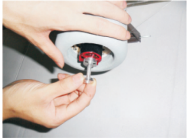
2. Installation gaskets.
