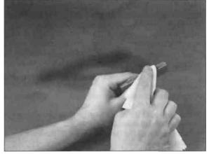
3. Excess epoxy will squeeze out of the seams between the joiners and must be removed before the epoxy is allowed to cure. Use a paper towel to remove the excess epoxy.
