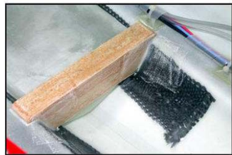
(above) Rear fuel tank support reinforced with fibreglass cloth.
