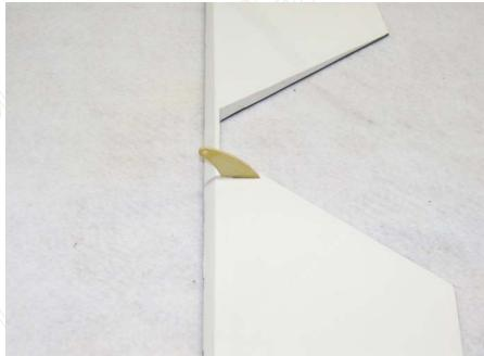
17. Slide the elevator onto the hinges in the stabilizer and secure with thin CA. Again a fresh bottle of CA and a fine glue tip work best here.
