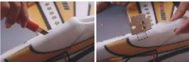
42. Insert the baldachin into the fuselage as shown .
