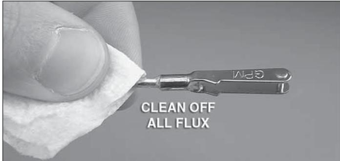
5. While the joint is still hot but after the solder solidifies use a clean, damp cloth to wipe the flux from the joint before it hardens. Flux is corrosive and must be thoroughly cleaned from the joint.
