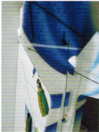
Same way to install hinge on rudder.
