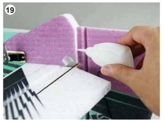
Glue the rudder in place as shown.
